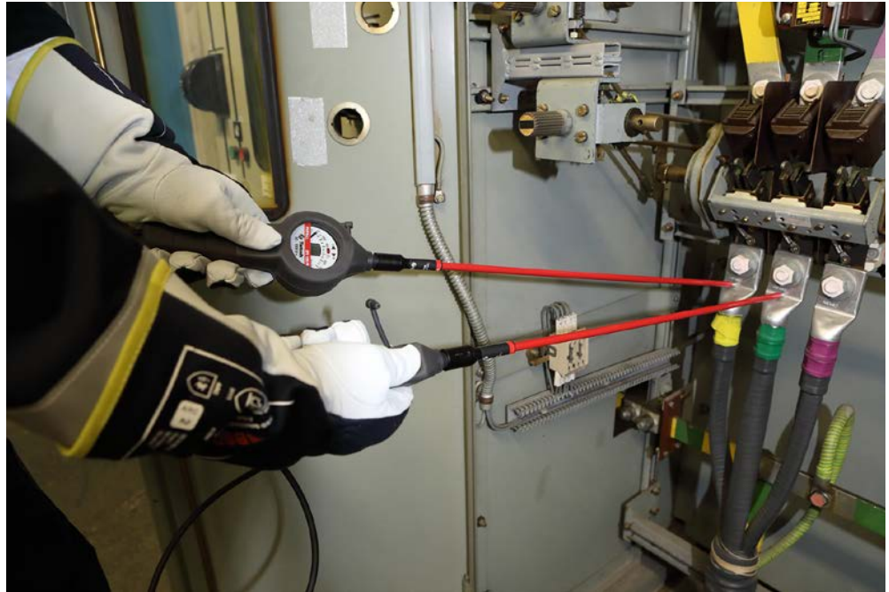
Fig. A 5-22 Determining a voltage-free state
