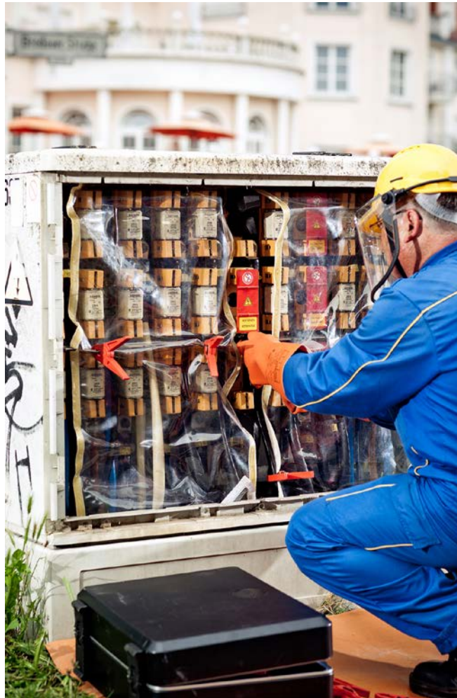
Fig. A 6-3 Working on a cable distribution cabinet: k_T = 1.5
