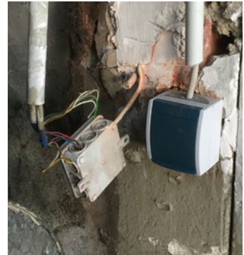
Abb. 6 Defekte Installation
